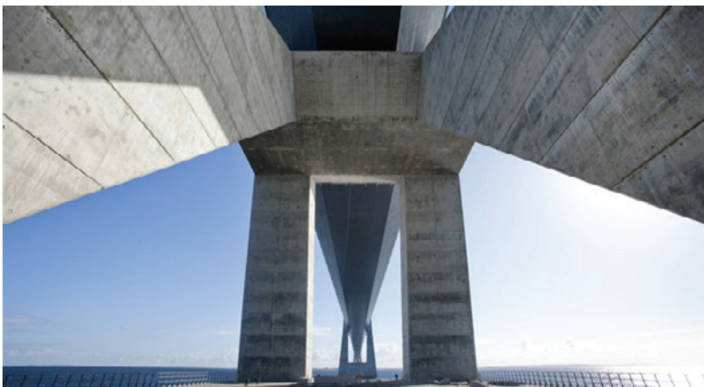
Project realized by Luigi Cividini Spa
