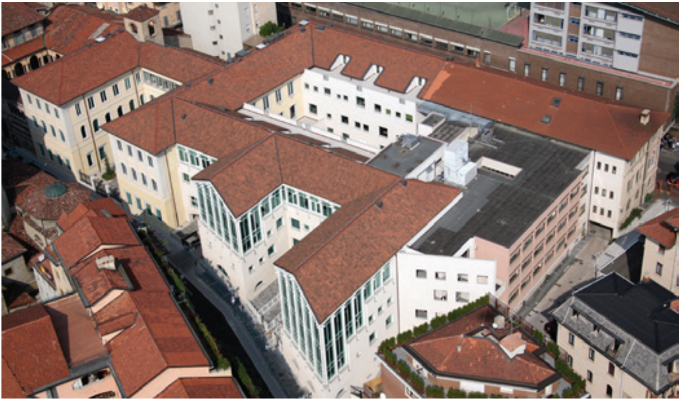
Project realized by Luigi Cividini Spa
